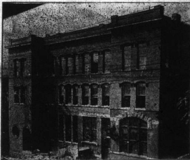
THE BIBLE SCHOOL BUILDING
