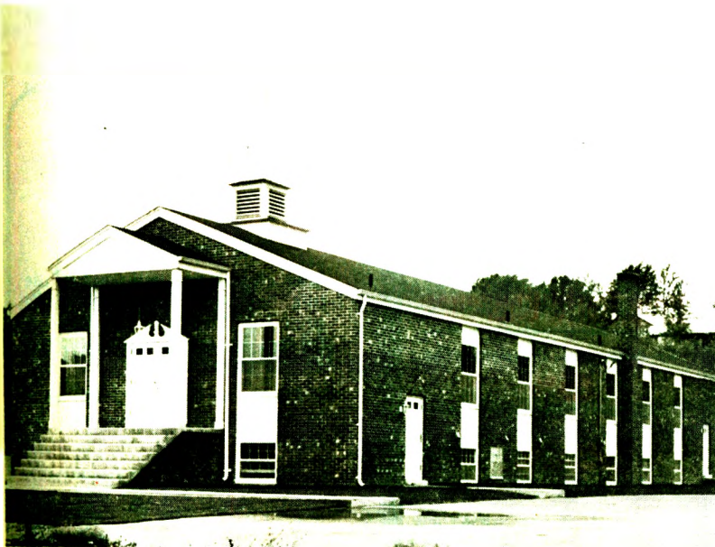
THE NEW NORTH HILLS CHURCH, Port Huron, Mich., was dedicated by Dr. Edward Lawlor in November. The church is located on seven and one-half acres just outside Port Huron. The colonial structure has a sanctuary seating 250. Valued at $150,000, it was built at a cost of $75,000. The church, organized four years ago, now has a membership of 83 with 135 attendance average in Sunday school. Pastor is C. Allen Henecke.
